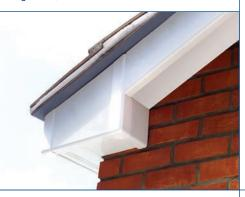
**Box End Detail 3:** Mammoth Board fascia, bargeboard, and box end cut from a section of fascia.
