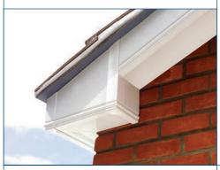
**Box End Detail 2:** Mammoth Board fascia, bargeboard, and box end cut from a section of fascia.
